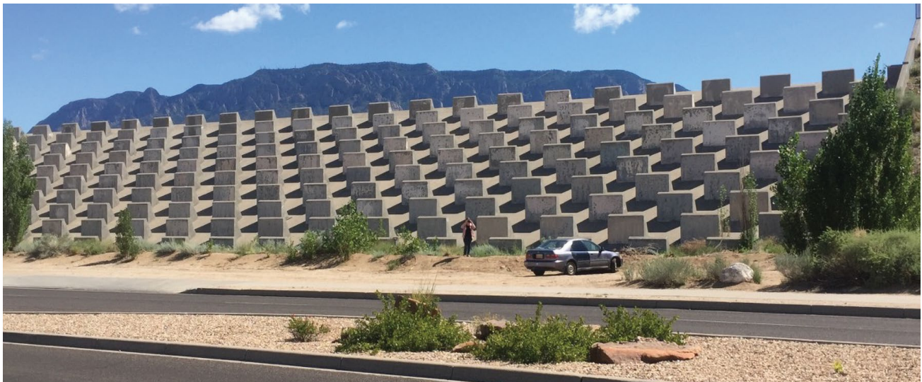
Figure 9.7. The emergency spillway for John Robert Dam, owned by the Albuquerque Metropolitan Arroyo Flood Control Authority. The spillway was designed to convey a flow of 23,600 cfs from a PMP storm. Photo by Bruce M. Thomson
